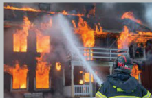
Fire & Smoke Damage
